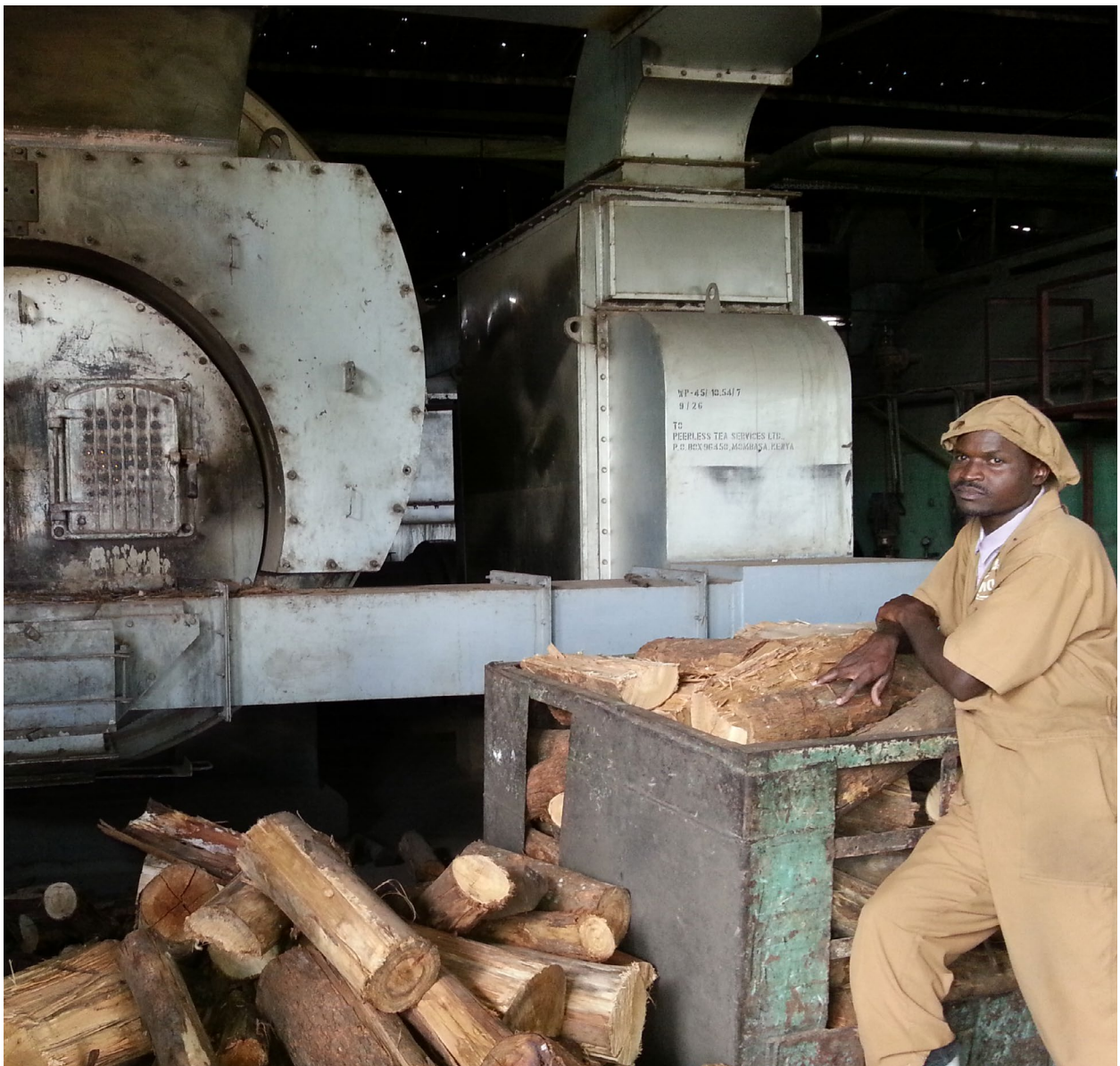
Steam generation by a boiler fired by measured firewood ▲
